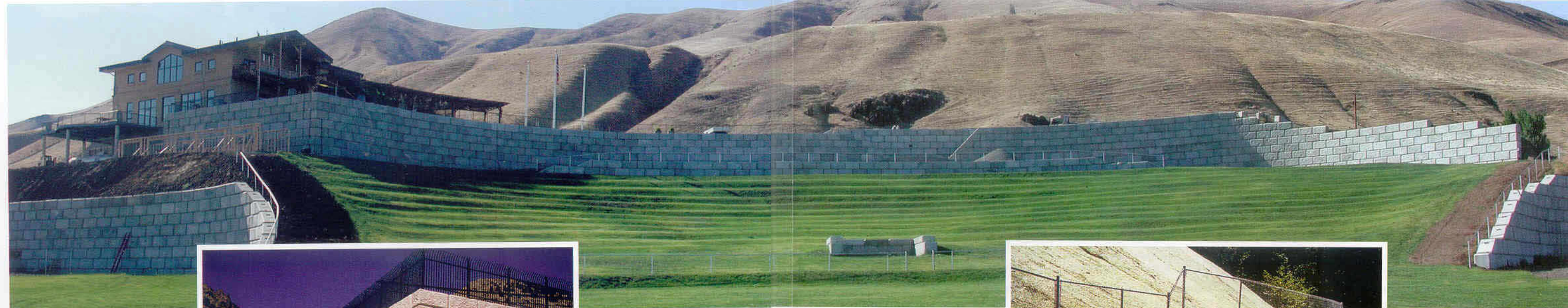
Maryhill Winery, Goldendale, Wa. Quarry Stone, MSE Design, supporting the outdoor visitor's wine tasting area and surrounding amphitheater.
