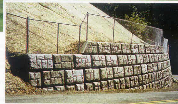
Thompson Road Slide Repair, Portland Or. Cut stone, wall reinforces the toe of a 1.5 to 1 back slope with a steel fence catchment.
