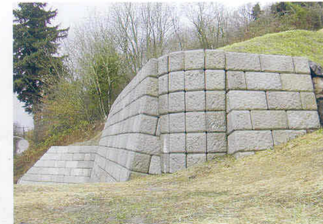
Evergreen Wall Project, Vancouver, WA. Quarry Stone, wedge blocks allow for a wall radius.
